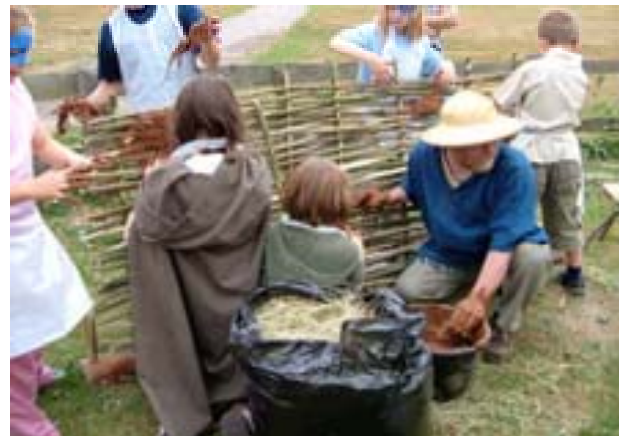
The wall nears completion
